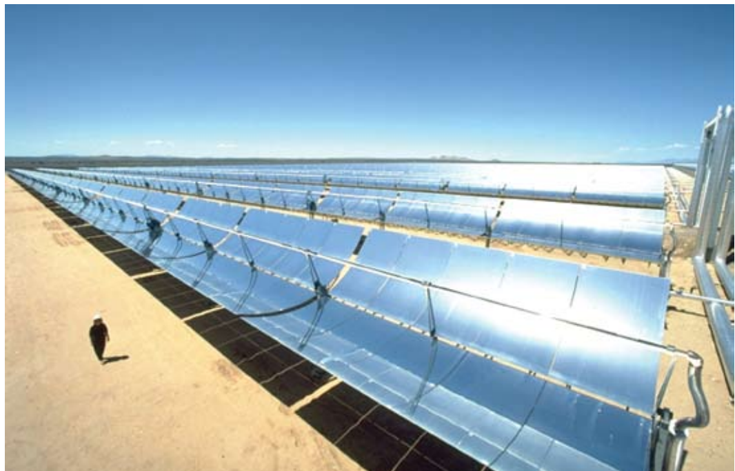
Parabolic trough concentrating solar power plants, such as this one in California, have the potential to generate large amounts of power in sunny areas of the Southwest and elsewhere. Credit: Gregory Kolb, Sandia National Laboratory
